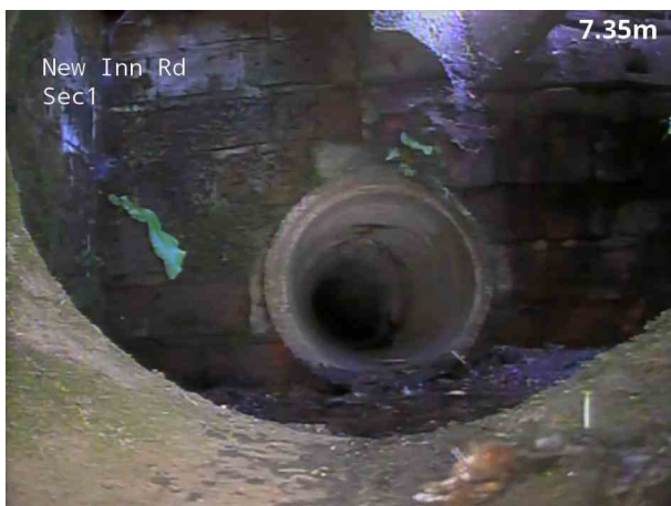
5, 00:00:47, 7.60 m Finish node, catchpit, reference: CP2
