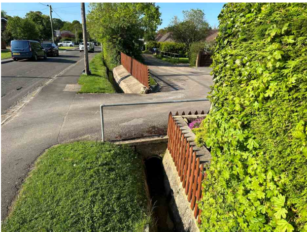
Ditch, East side of New Inn Rd
