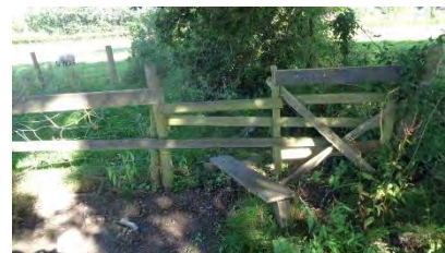
Broken Stile at eastern end
