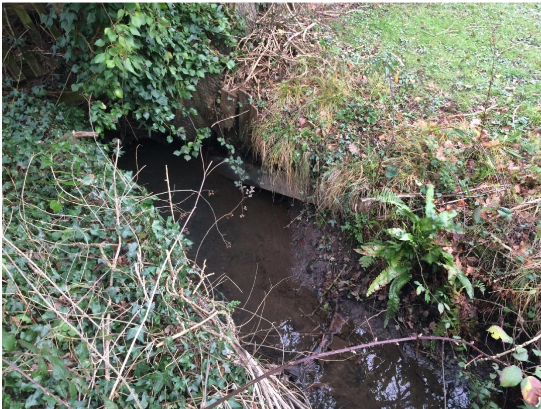
Image 4: Outfall of drainage system (suspected previous ditch) on east of Pollards Moor Road, flowing into watercourse that becomes Main River, facing south-east (Jan 2018)
