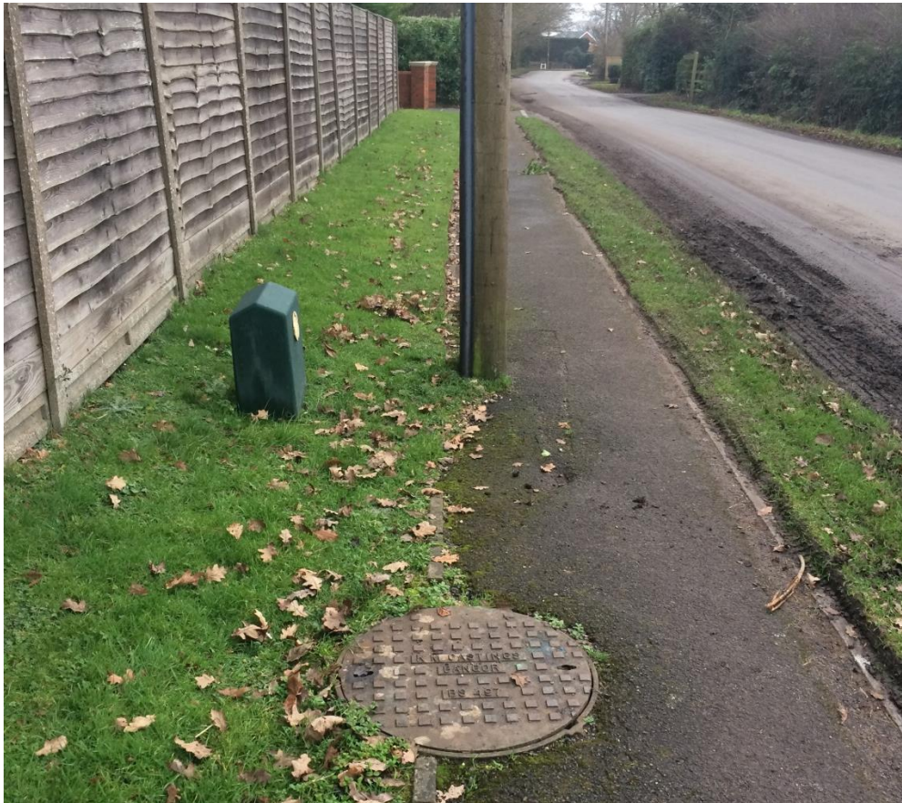
Image 2: Telegraph pole along line of surface water drainage system, east side of Pollards Moor Road at the north end, past Vicarage Lane, facing south-east (Jan 2018)
