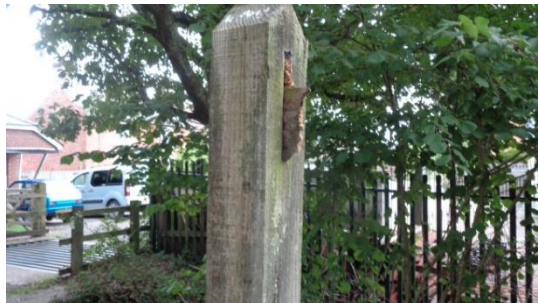
Broken Finger post at Cadnam end
