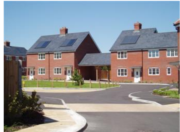
Community led housing Wickham
